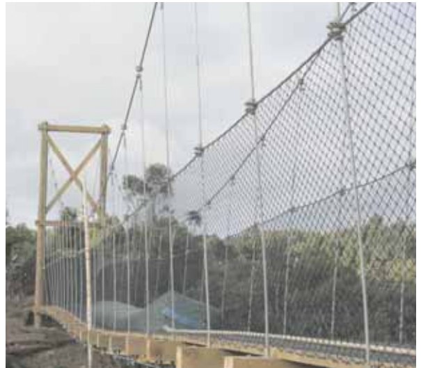
Load testing the bridge; credit DOC
