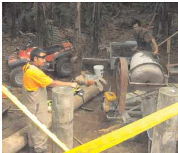
Community max workers undertaking track construction; credit DOC.
