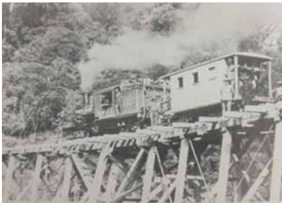
Climax loco on Goat Creek bridge, 1926
